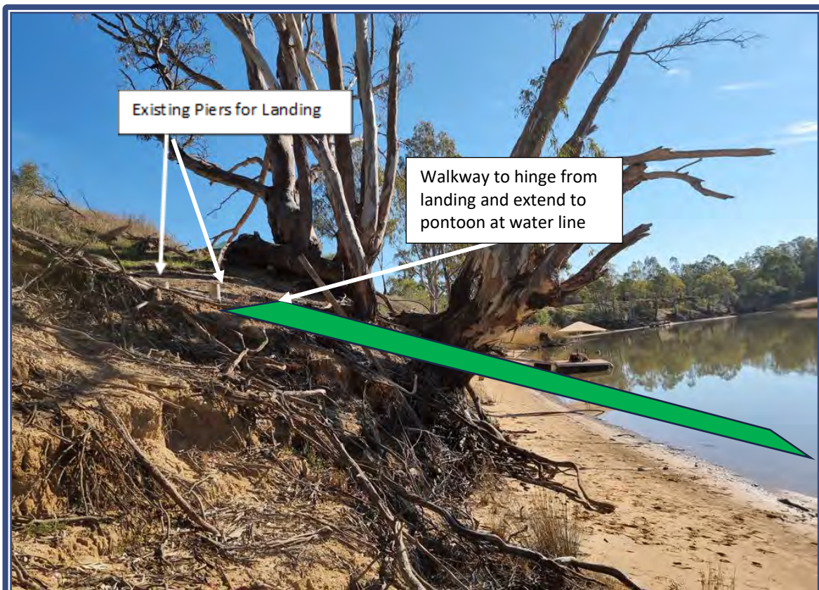
Figure 4-3 - Image showing landing location and hinge of walkway (Source: PRS) Note structure in background unrelated to this application)
